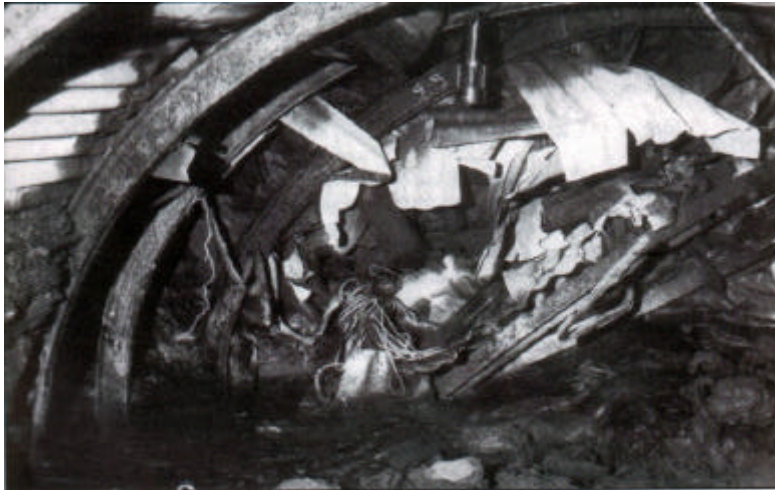
Fig 2 The aftermath of the inrush of water into Lofthouse Colliery in 1973. The picture shows the blockage in the South 9B District main gate. All the telephones in the large section of the mine involved were on a one-party-line extension which became hopelessly blocked. (Crown Copyright, HMSO, loaned from National Coal Mining Museum for England).
